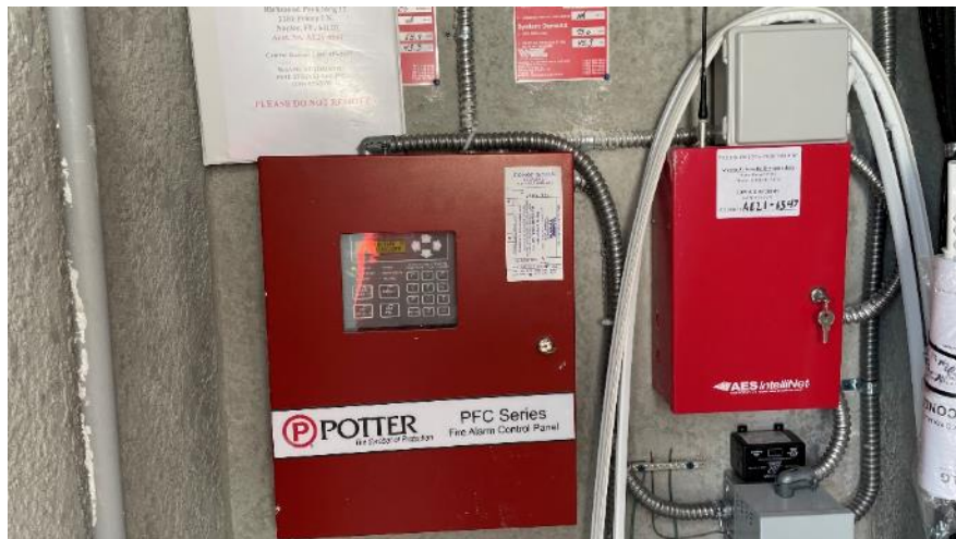
Photograph 3: Fire Alarm Control Panel located within air-conditioned space
