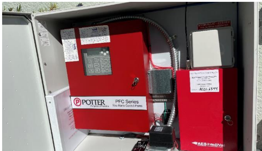
Photograph 4: Fire Alarm Control Panel located on side of condominium building
