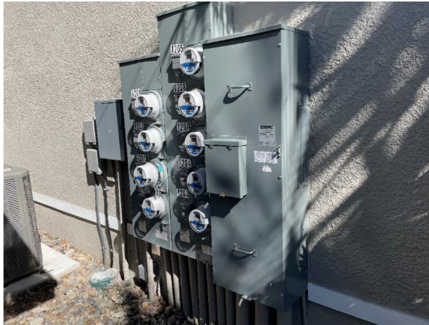
Photograph 6: Main electrical panel and meter bank at 2281 Priory Lane
