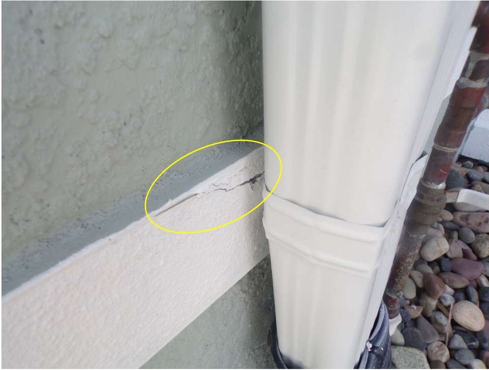
View of typical stucco damage observed.
