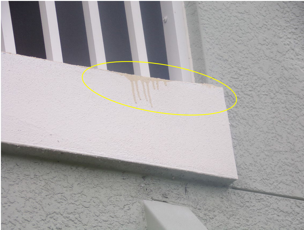
View of typical paint drippage.
