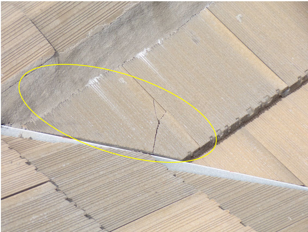
View of typical shattered roof tile.
