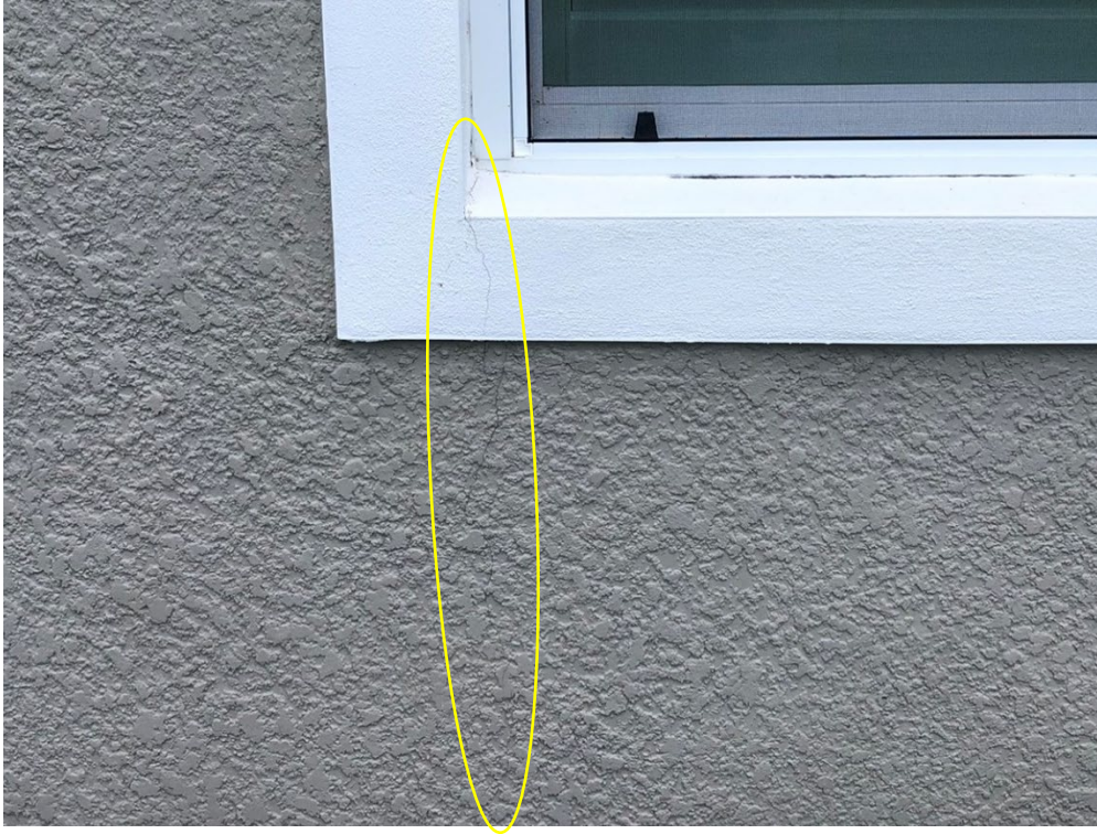
View of typical stucco cracking observed.
