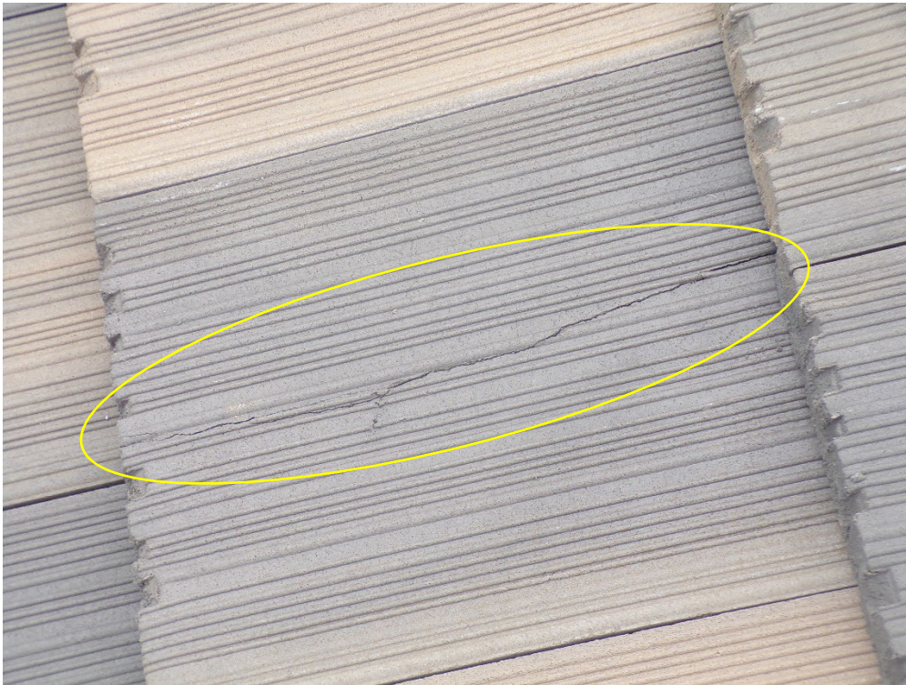
View of shattered roof tile.
