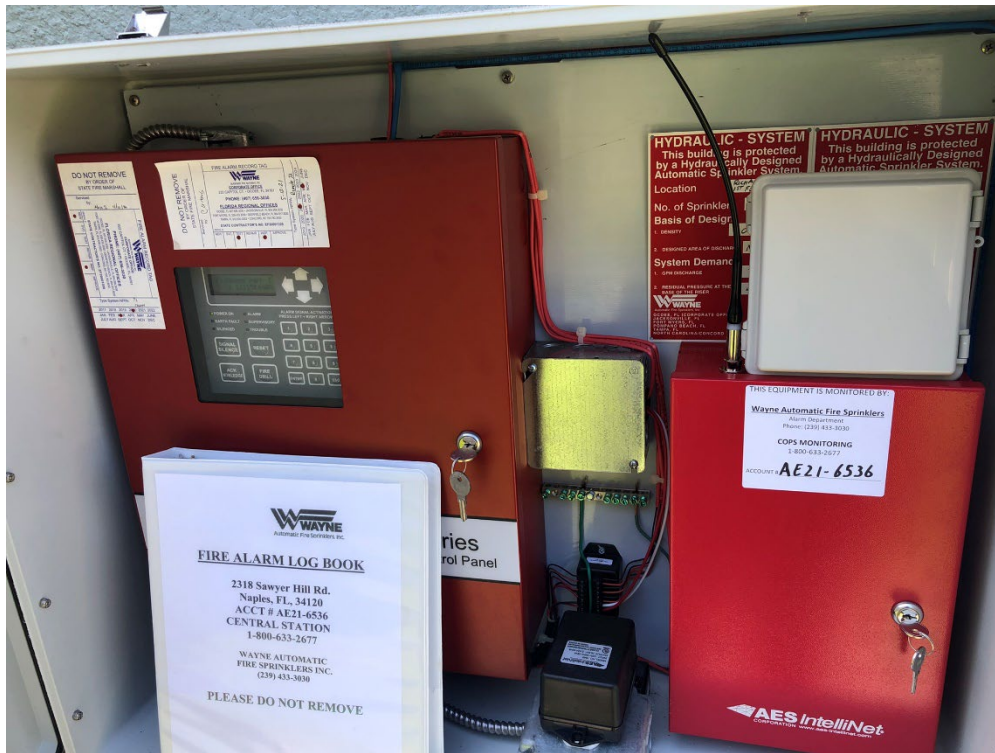
View of typical FACP controller, with expired inspection tag.
