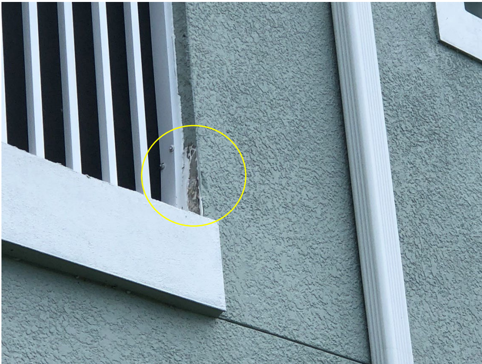
View of damaged stucco on building 2327.
