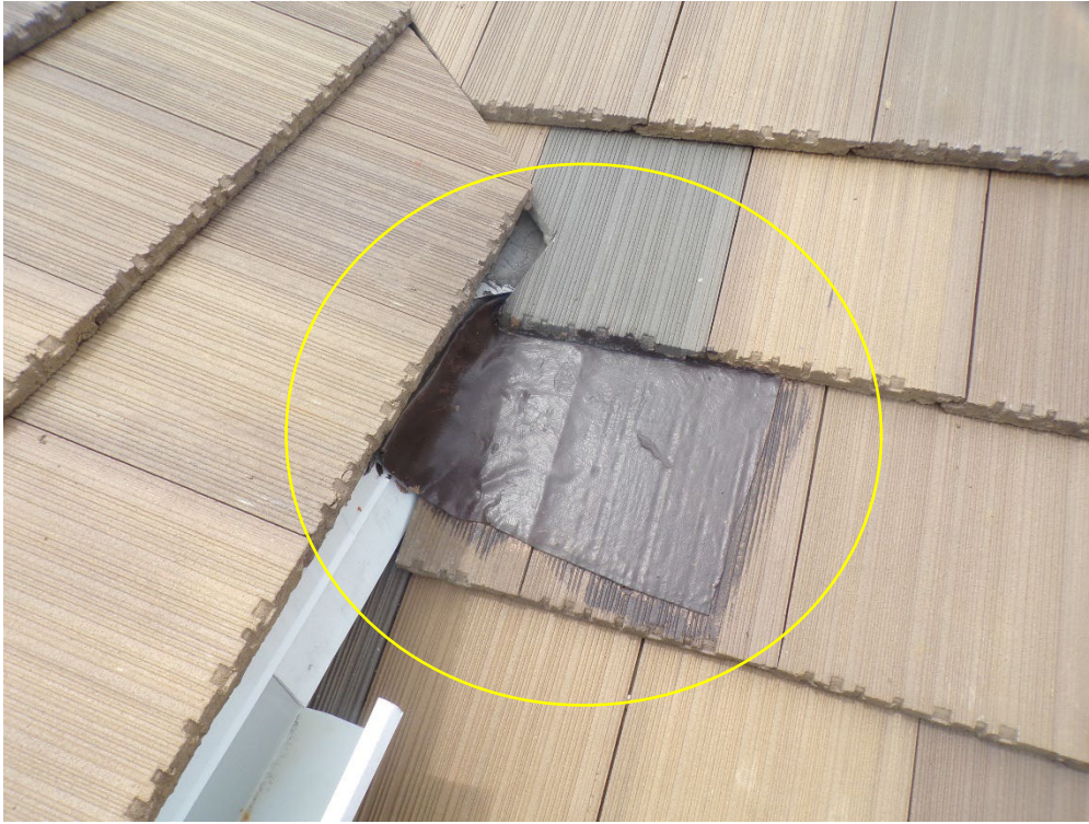
View of incomplete flashing metal installation.
