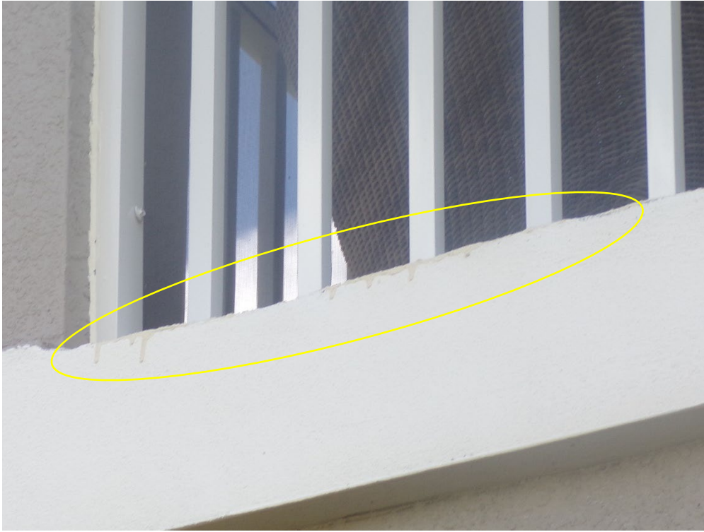
View of typical paint dripping.
